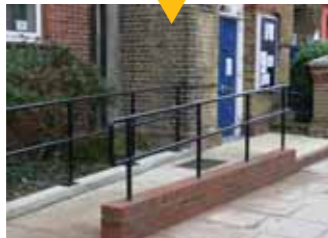
Ramp and hand rail were added to the entrance of the centre.
