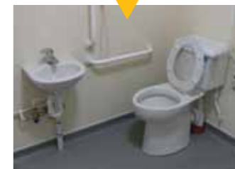
St John's Community Centre – disabled toilets
