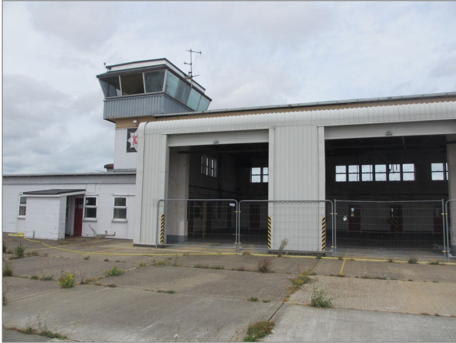
Figure 13: Dilapidated Rescue & Fire Fighting Facility
