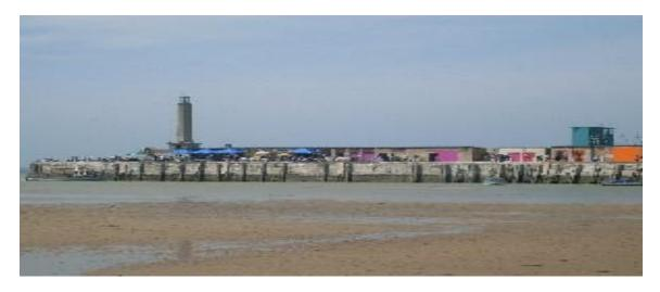
Margate Harbour is a small drying site which is protected by a large stone breakwater, the Harbour Wall itself being constructed as a series of compartments filled with rubble and shingle and has now firmly withstood the fury of the sea for 186 years
