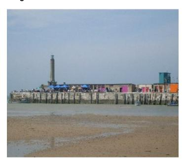
Margate Harbour is a small drying site which is protected by a large stone breakwater, the Harbour Wall itself being constructed as a series of compartments filled with rubble and shingle and has now firmly withstood the fury of the sea for 186 years
