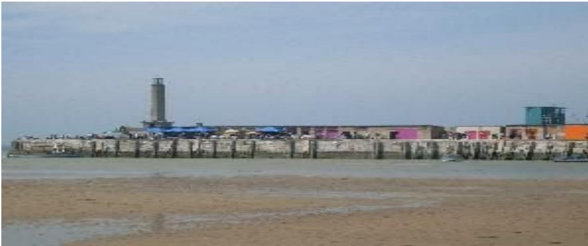
Margate Harbour is a small drying site which is protected by a large stone arm, the Harbour Wall itself being constructed as a series of compartments filled with rubble and shingle and has now firmly withstood the fury of the sea for almost two centuries.
