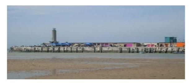
Margate Harbour is a small drying site which is protected by a large stone breakwater, the Harbour Wall itself being constructed as a series of compartments filled with rubble and shingle and has now firmly withstood the fury of the sea for almost two centuries.
