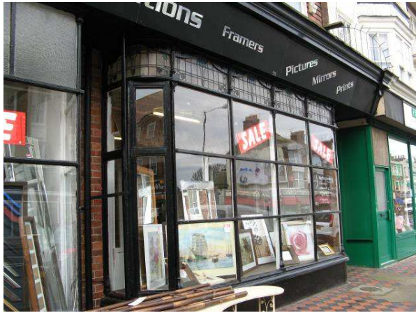
Historic shopfronts in Northdown Road
