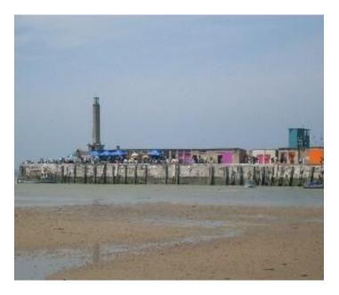
Margate Harbour is a small drying site which is protected by a large stone breakwater, the Harbour Wall itself being constructed as a series of compartments filled with rubble and shingle and has now firmly withstood the fury of the sea for 186 years
