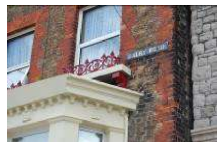
Dentil moulding to canted bays stone corbels and cast iron window guards
