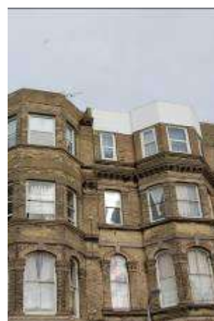
Re-built upper storey lacking historic detailing
