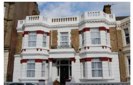
Brick built with highly decorative stucco detailing
