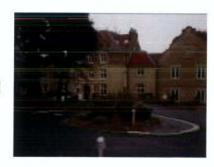
The core of this large property dates from 1795 however it has been extended in the late 19<sup>th</sup> century. Constructed of stock brick the main block is rendered with flint extensions to the sides and plain tiled roofs. The front elevation, which is viewed from London Road, consists of three storeys with a hipped roof, rendered from the first to the ground floor
