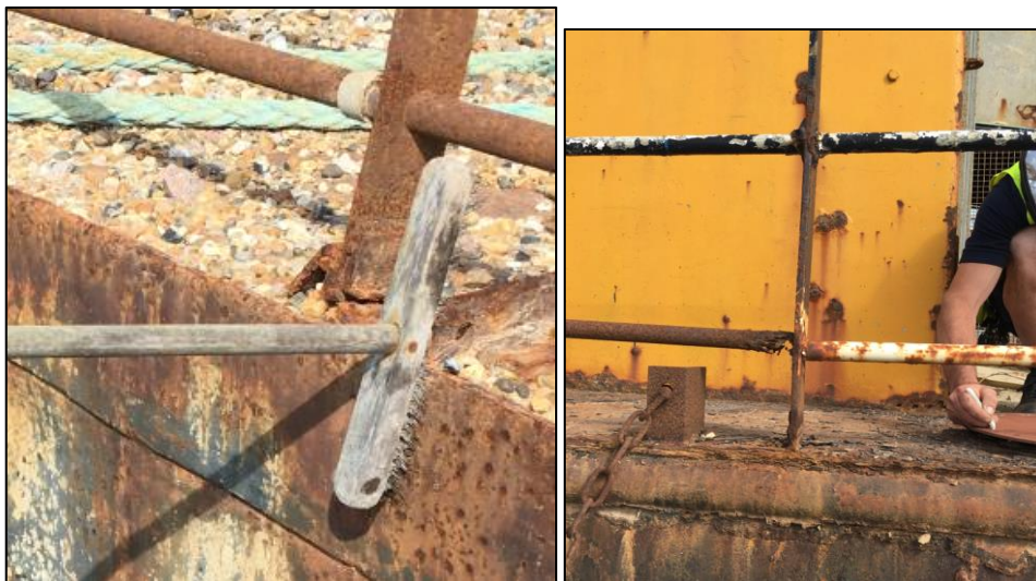
Figure 39 Edge Protection Handrails
