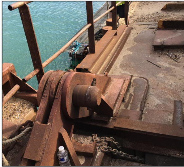
Figure 24 Barge Articulated Hinge Connection (Northside)
