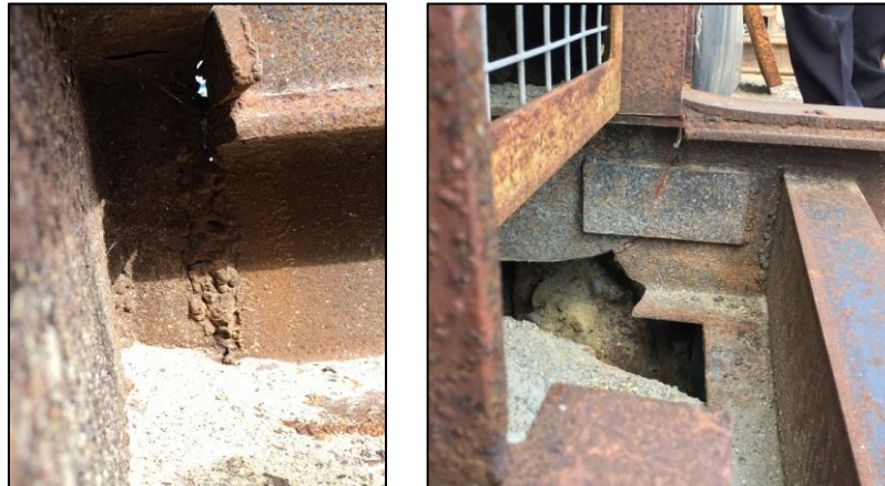
Figure 27 Hinge Connection Fracture Repair (Northside)
