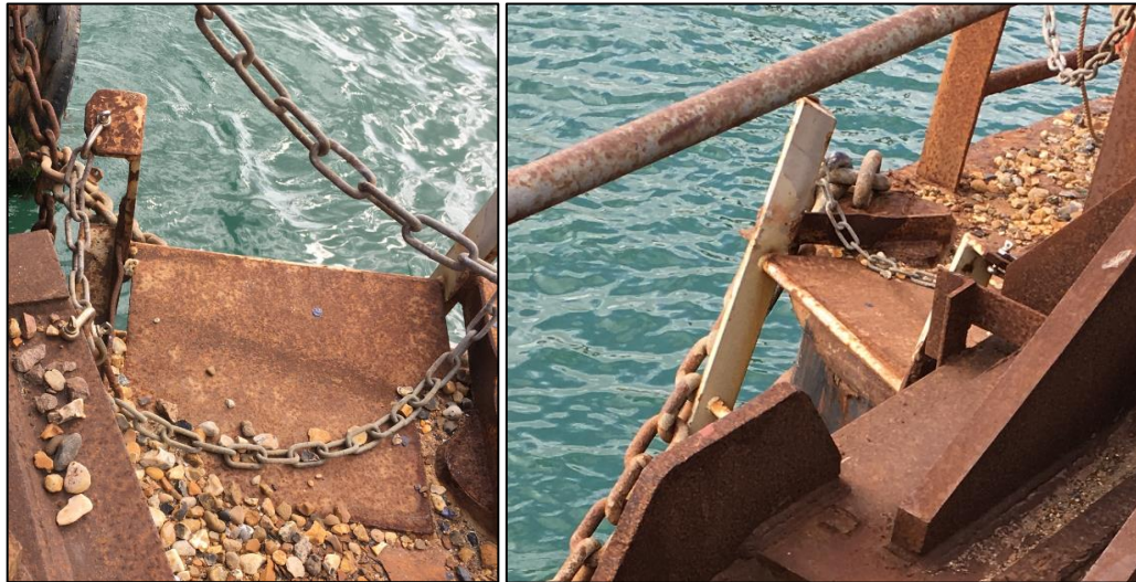
Figure 37 Emergency Access Ladder Connection (Southside)
