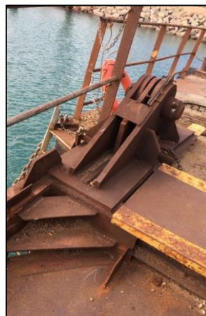
Figure 28 Barge Articulated Hinge Connection (Southside)
