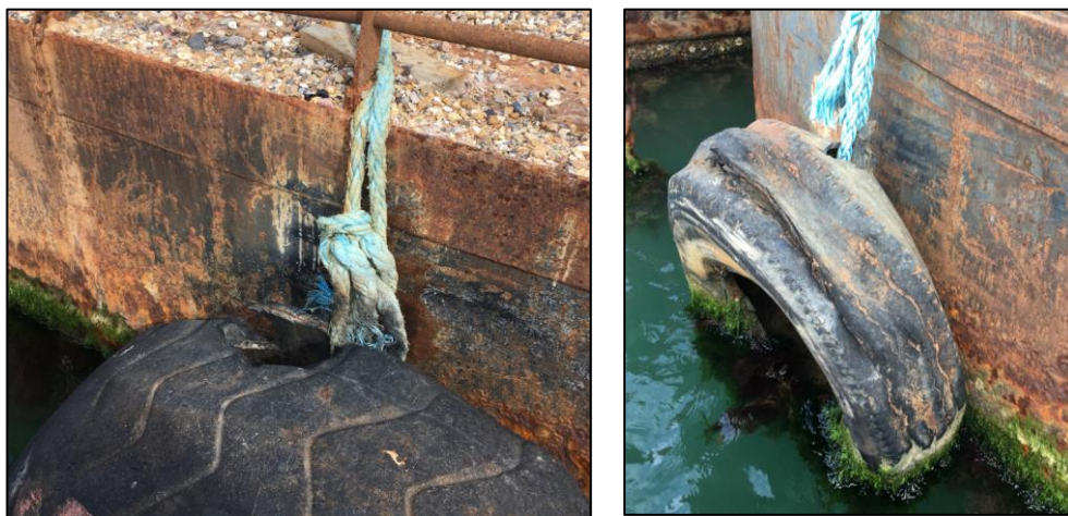
Figure 41 Fender Decay (Rope Support)
