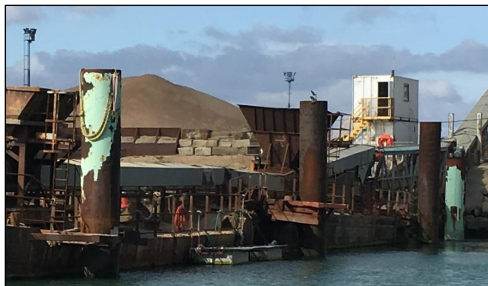
Figure 31 Barges Guide Piles
