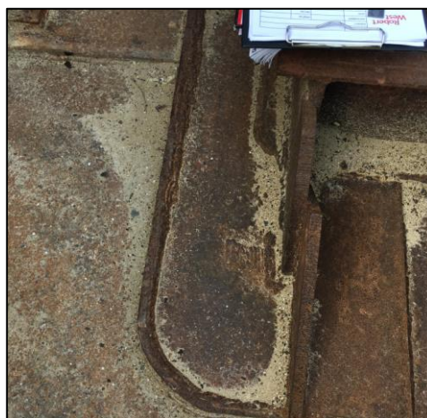
Figure 26 Hinge Connection Additional Plate (Northside)
