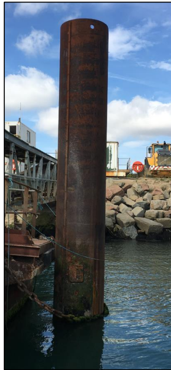
Figure 30 Barge No.1 Guide Pile (NW Corner)
