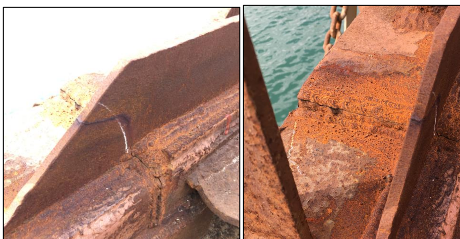
Figure 29 Hinge Connection Fracture (Southside)
