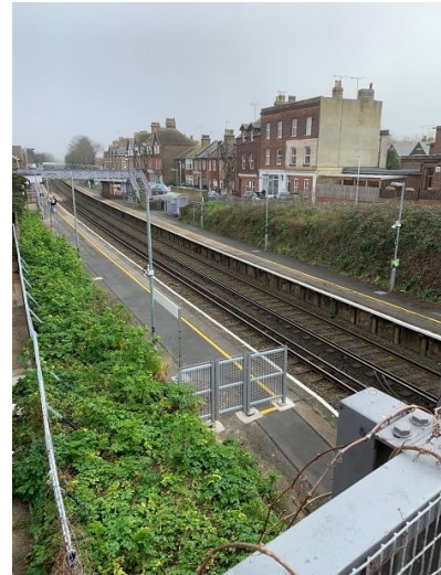
Figure 19-1 Westgate Railway Station
