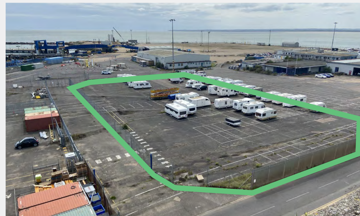
Site A & B, view from cliff top.
